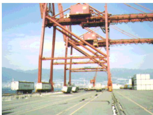
Fig. 2.7 Seaward lateral movement of rail foundation and differential settlement of rails [1995 Hyogo-ken Nanbu (Kobe) earthquake, Rokko Island]
