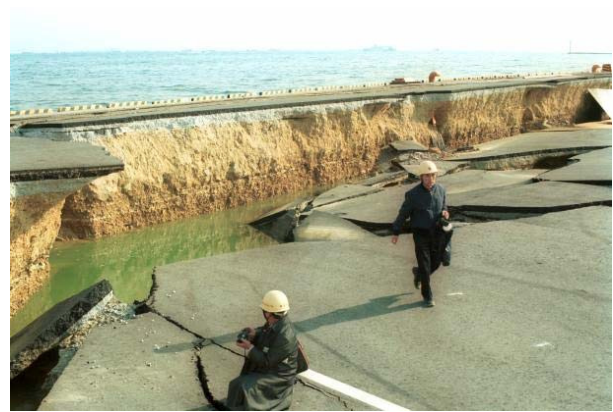
Fig. 2.5 Seaward displacement and tilting of quay-walls during the 1995 Hyogo-ken Nanbu (Kobe) earthquake
