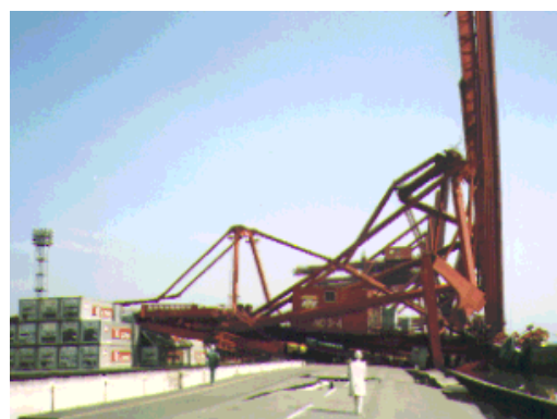
Fig. 2.8 Crane total collapse. Various damages to other cranes like plastic hinges and bending of their members [1995 Hyogo-ken Nanbu (Kobe) earthquake, Rokko Island]
