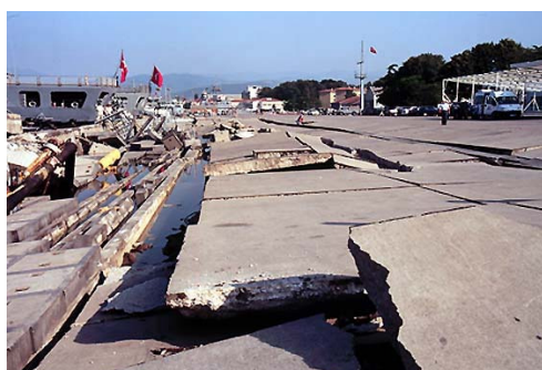
Fig. 2.2 Damaged quay walls at Golcük navy base during the 1999 Kocaeli earthquake
