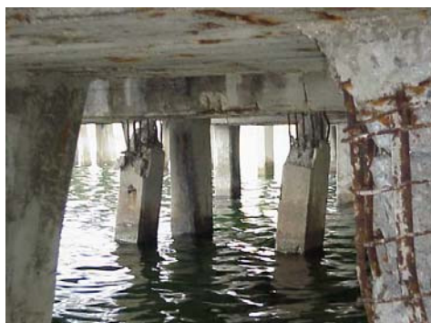
Fig. 2.1 Damage to waterfront structures and supporting piles during the 1999 Kocaeli earthquake
