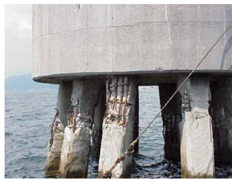
Fig. 2.1 Damage to waterfront structures and supporting piles during the 1999 Kocaeli earthquake
