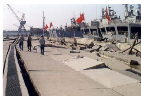
Fig. 2.2 Damaged quay walls at Golcük navy base during the 1999 Kocaeli earthquake
