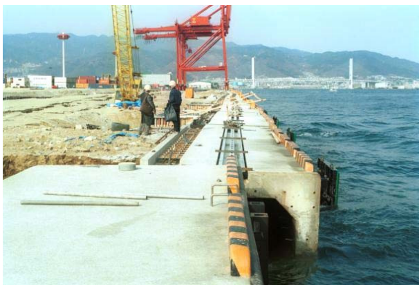
Fig. 2.5 Seaward displacement and tilting of quay-walls during the 1995 Hyogo-ken Nanbu (Kobe) earthquake
