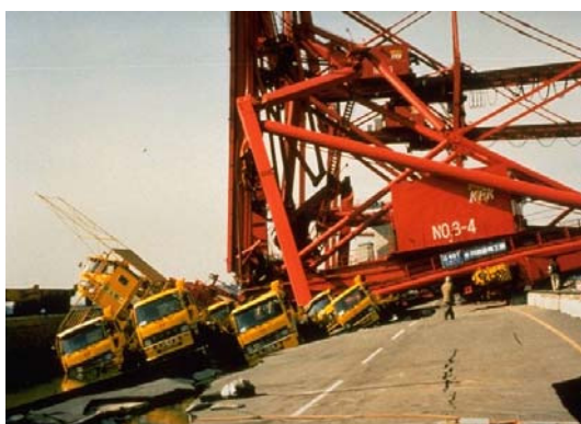
Fig. 2.9 Crane damage during the 1995 Hyogo-ken Nanbu (Kobe) earthquake
