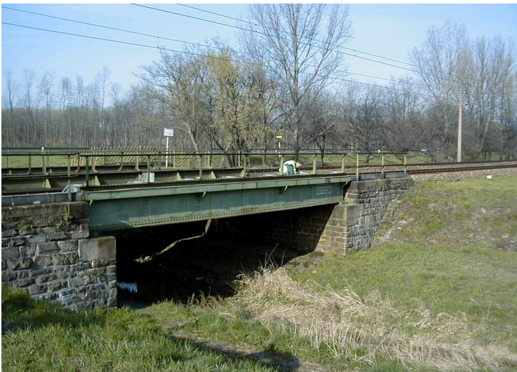
Fig. 2 Rohrbachbrücke in Austria built 1903
